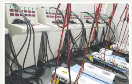
Heat Run Test
